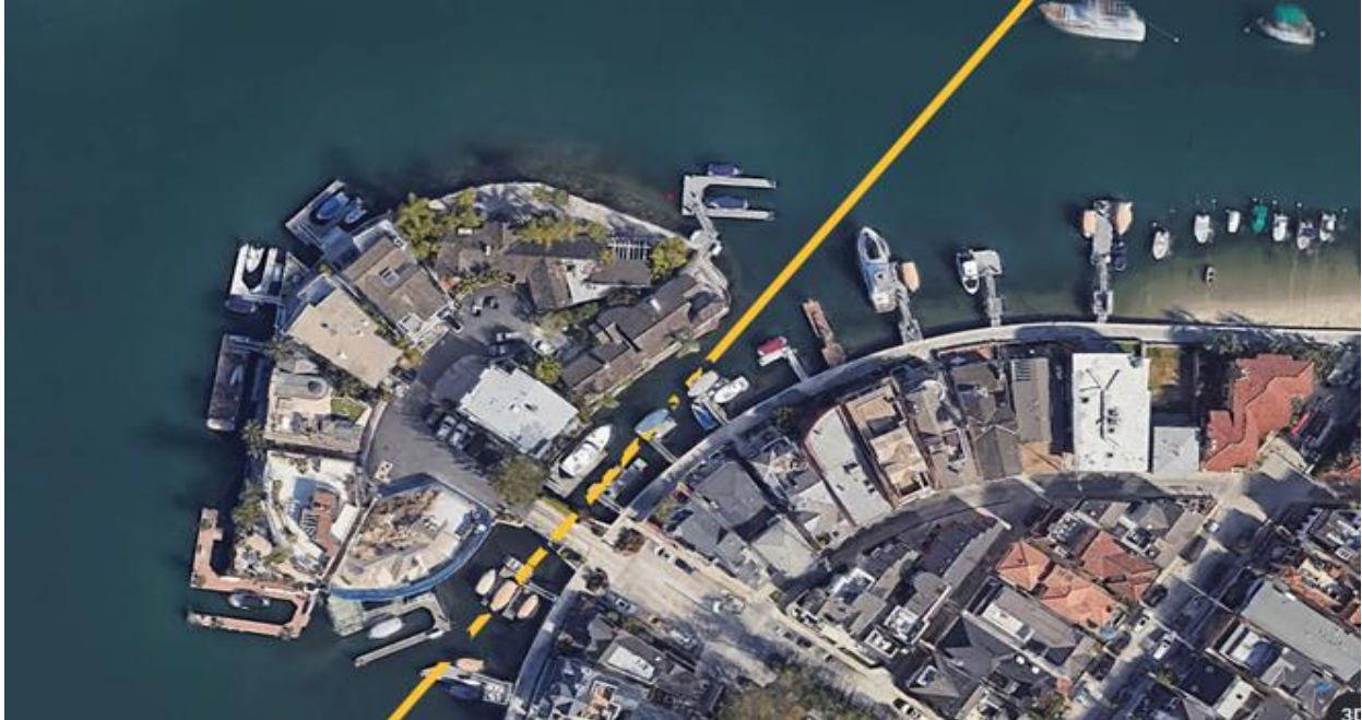
FIGURE 5: WATERS WAY BRIDGE (No. 55C-0265) OVER NEWPORT BAY. YELLOW LINE MARKS THE BOUNDARY BETWEEN COLLINS ISLAND (TO THE WEST) AND BALBOA ISLAND (TO THE EAST) (GOOGLE EARTH 2023).
