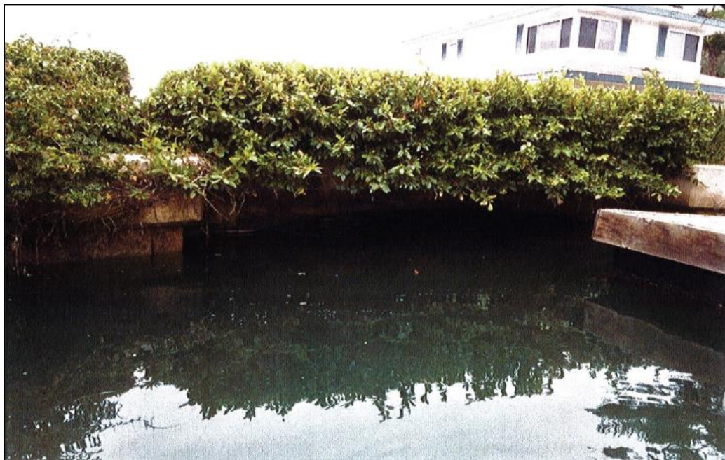
Photograph 5: Overview of the north side of the bridge in 2017, view southwest (Caltrans 2017).
