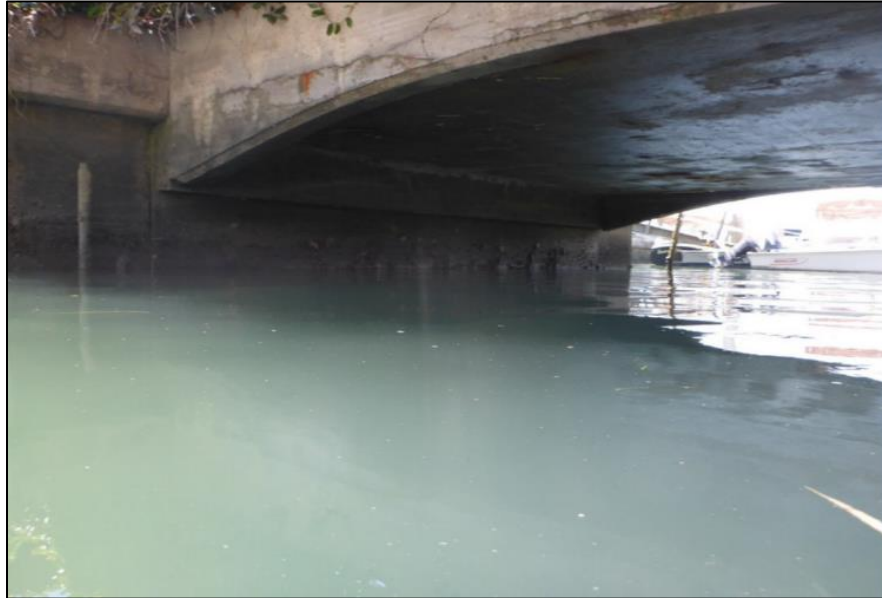
Photograph 6: Underside view of the bridge in 2018 looking north (Caltrans 2018).
