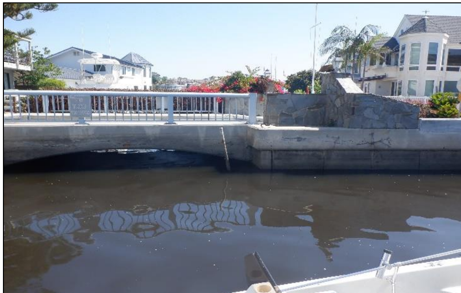
Photograph 3: Overview of the south side of the bridge where it connects to Balboa Island. View northeast, August 22, 2023.
